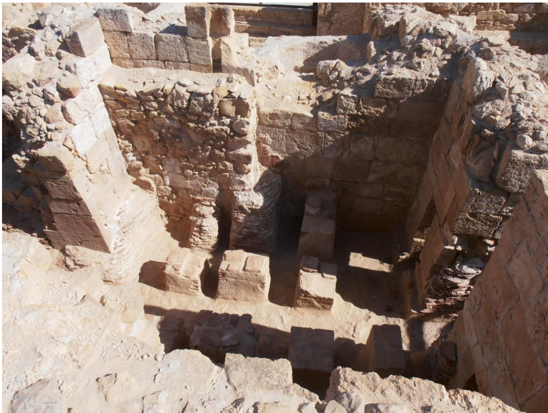
Fig. 13. Hypocaust heating system at Mamshit. Photo courtesy of Dominik Elkowicz.
