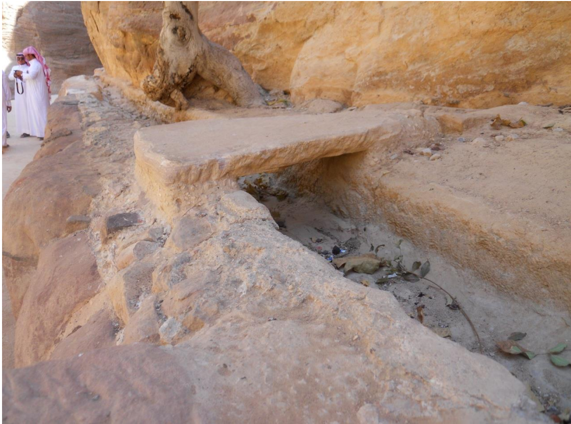
Fig. 20. The Siq aqueduct covered by stone slabs.
