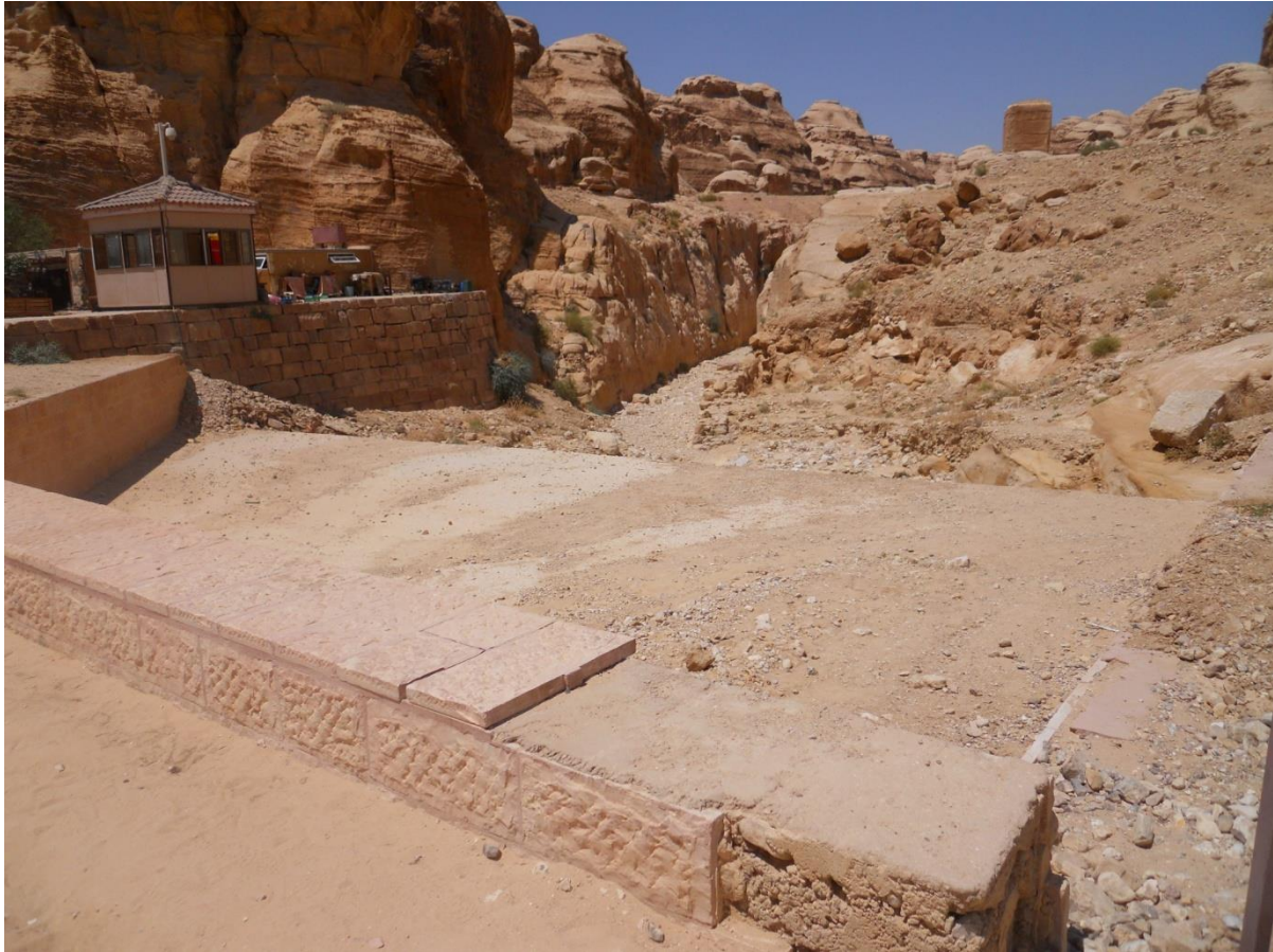
Fig. 26. Settling basin at the entrance to the Siq
